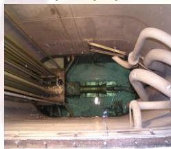
Zone 1 - dismantling of reactor internal systems loop equipment
